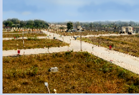
Cement Concrete Road
