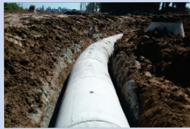
Concrete Pipeline for Drainage
